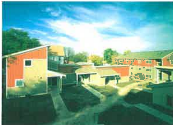
...St. Philip's Gardens After Rehabilitation
